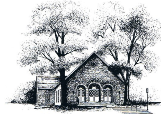
Timber Ridge "Old Stone" Presbyterian Church c. 1755
